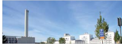
Operational renewable energy plant in Hammarby, Stockholm
