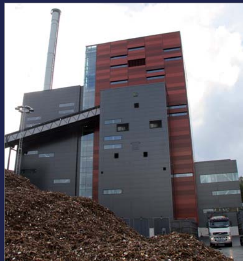
Power plant with fuel stocks
