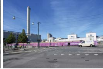
Plant and adjacent housing site under construction
