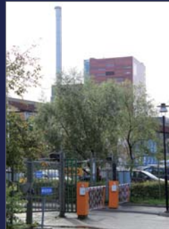
Sodertalje power plant
