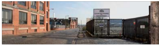
View of the outline shape of the plant from Salamander Street
