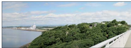
View of the outline shape of the plant from Forth Road Bridge (north)
